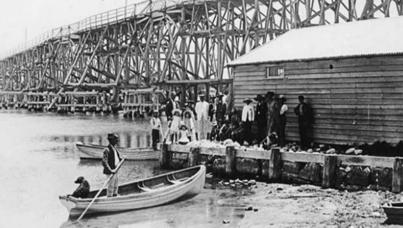
High Level Bridge 1866: the first Fremantle bridge was built out of timber by convict labour 1863-7, and was officially opened 2 October 1867. (Hitchock: 52)
