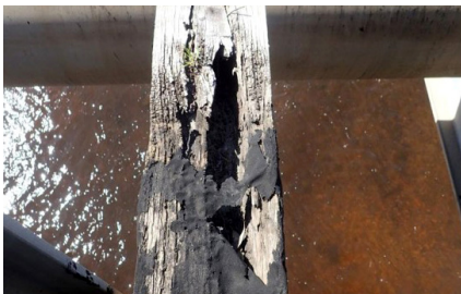
Span 3 LHS top of bearer 5.
