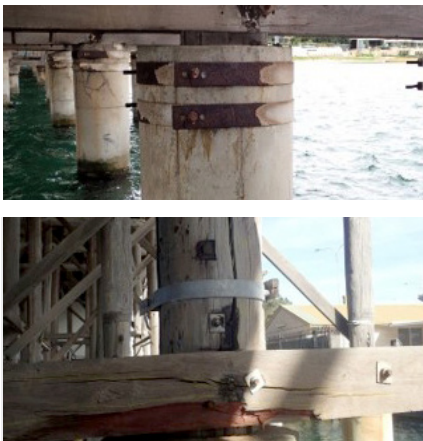
Cracks in the concrete protection jacket allowing sand to leach out
