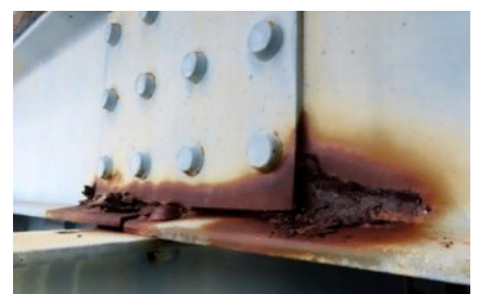
Span 17 stringer 11 loss of section.
