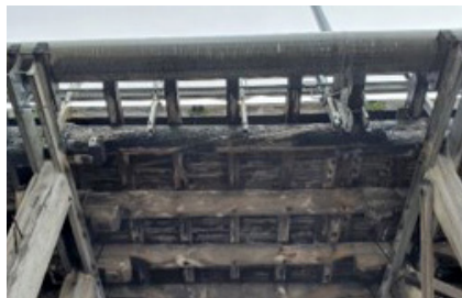
Deck reinforcing and lack of shelter to outside stringers.
