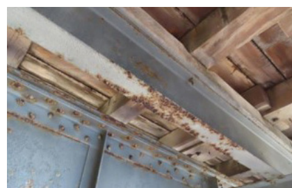
Main girder, transverse support and stringer.
