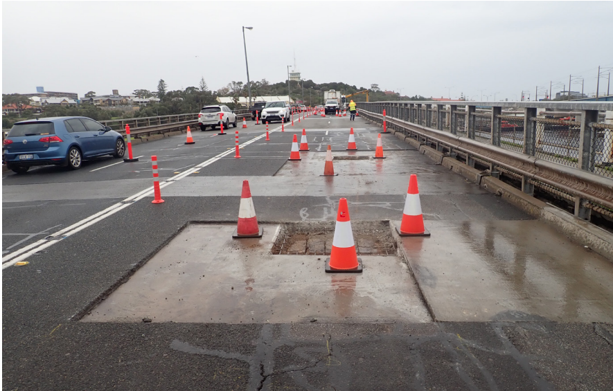
Sections of the road surface removed.
