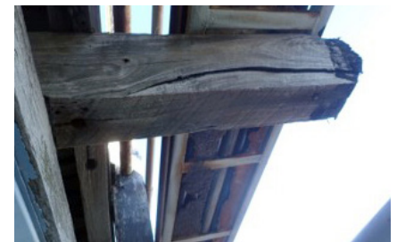
Tray below footpath.
