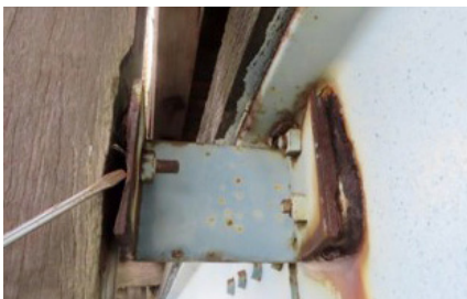
Corrosion of bolted connections.
