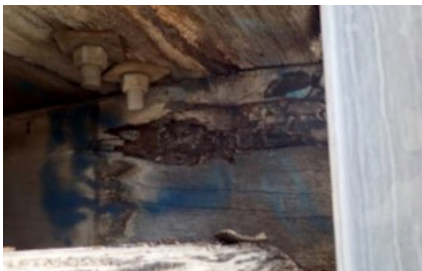
Timber at the location of bolts securing the guardrail post to the deck.
