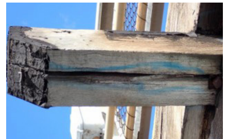
Weathered timber - split bearer and corbel.
