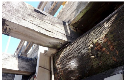
Weathering of outside stringer.
