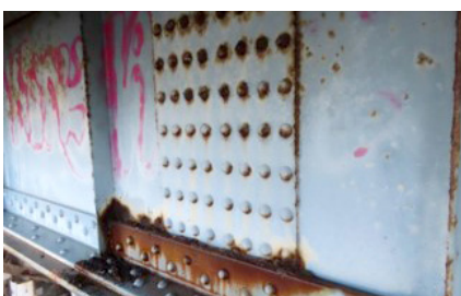
Corrosion of bolts and rivet heads.
