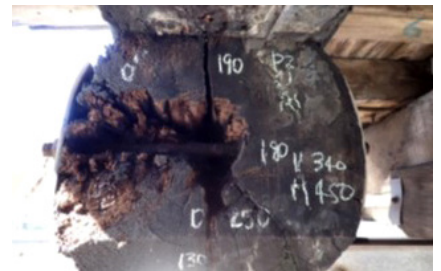
Weathered split timber from corroding bolts.
