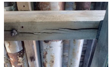
Pipes below footpath.
