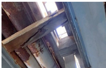
Deterioration of bolt connections.
