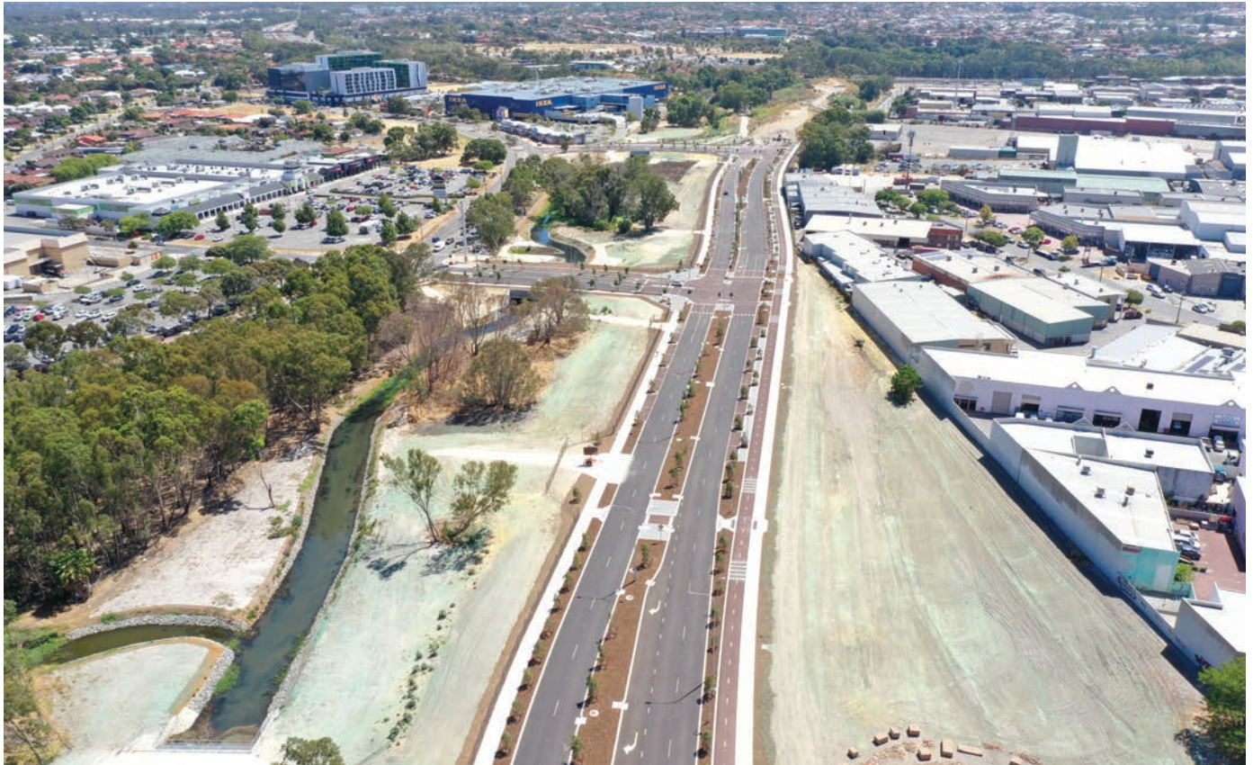
Stephenson Avenue Extension Project Phase 1 - February 2022
