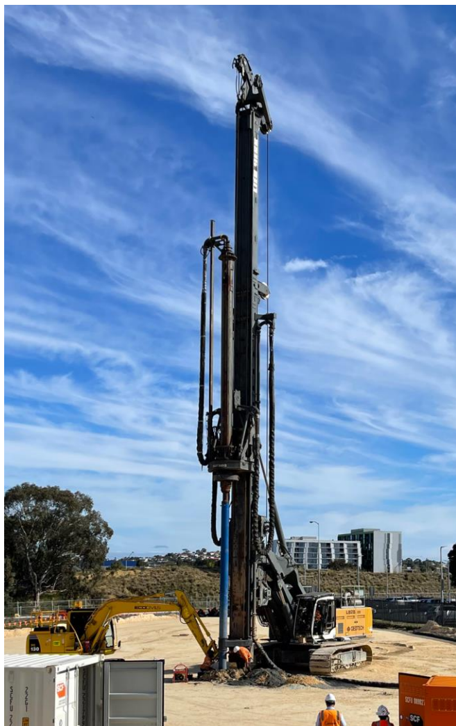
The piling rig being inspected prior to commencing CMC works
