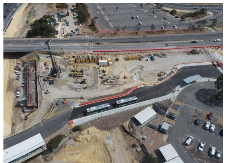
Construction of the casting bed at the Stirling Station bus interchange.
