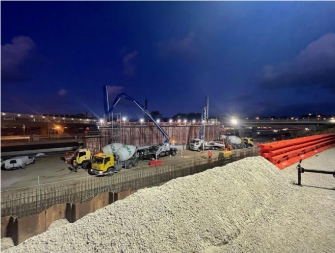
Concrete trucks pumping into the pier.
