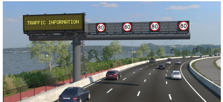
Smart Freeway's new Lane Use Management System will open and close lanes during a traffic incident and provide real-time information to road users
