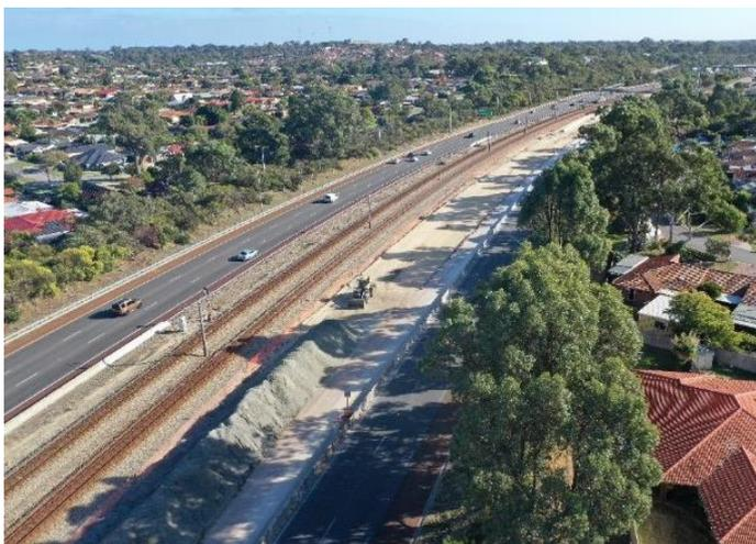
Figure 2: Pavement works to create the new freeway lanes
