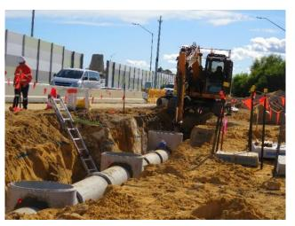
Figure 1: Drainage works below Burns Beach Road entry ramp
