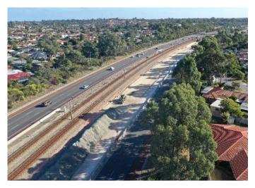
Figure 2: Pavement works to create the new freeway lanes
