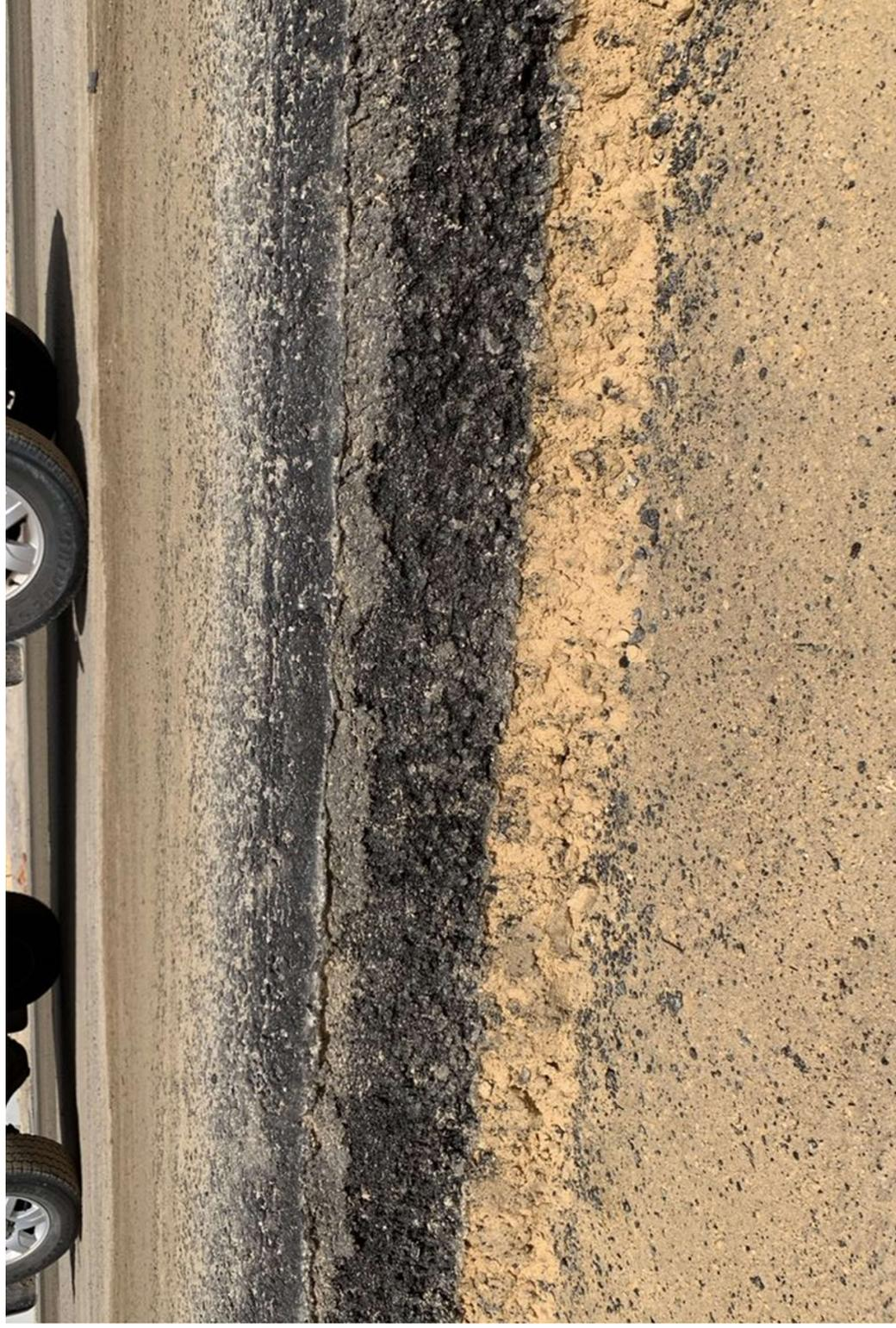
Representation of the layers required to construct the Mitchell Freeway southbound widening. Each layer requires compaction
