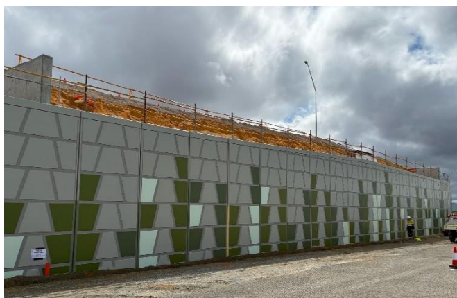
Image (above): Reid Highway / Altone Road bridge abutment walls.
