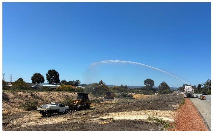
Above image: Works underway near Reid Highway and Altone interchange.
