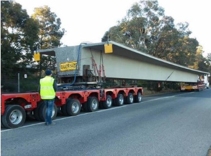
*Tee-roff beams up to 40 m long will be installed at the Muchea South Road bridge.*
