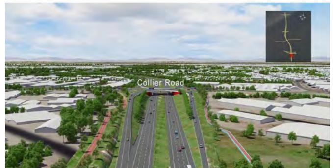
**Morley Drive** - there will be a roundabout at ground level, which will connect with a raised Tonkin Highway bridged over the roundabout. This is the first interchange of this type to be built in Western Australia and offers significant safety benefits.
