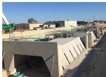
Precast trapezoidal underpass structure at Collier Road/Tonkin Highway
