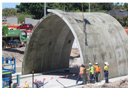
A three-pin self-supporting arch system is being used at the Morley Drive/Tonkin Highway pedestrian underpass
