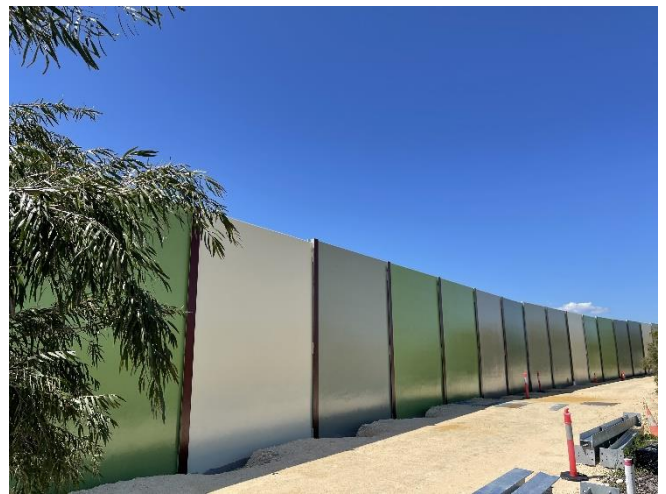
Panel and post noise wall on Manasota Approach
