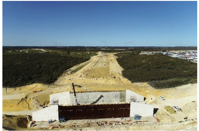
Romeo Road bridge over rail
