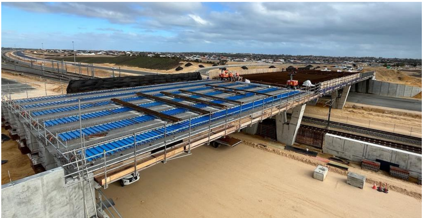
Lukin Drive interchange bridge
