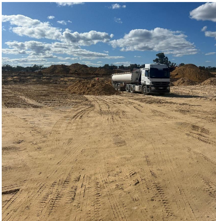
Fill transfer from METRONET
