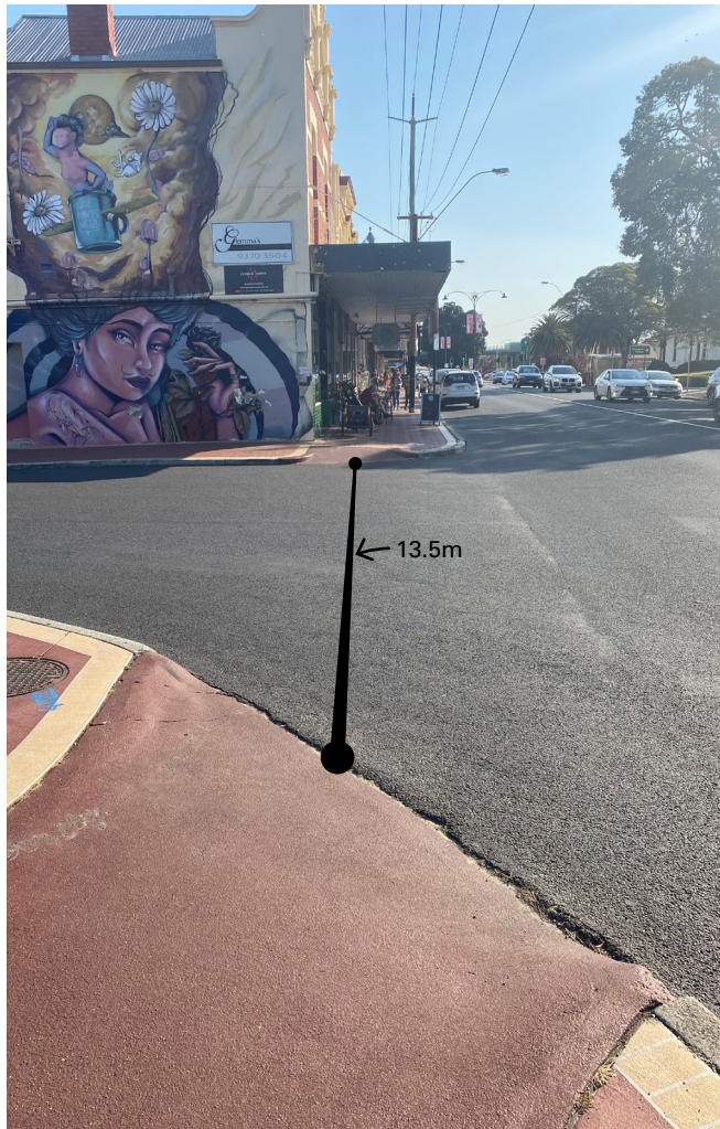
Distance over intersection too large (below 7m is preferred) Ninth Avenue
