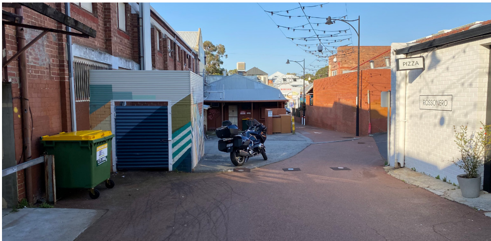
Sharp angles and reduced visibility means people driving do not travel at speeds above 10km/h. This is a safe place for people walking from a traffic perspective, but more surveillance is needed
