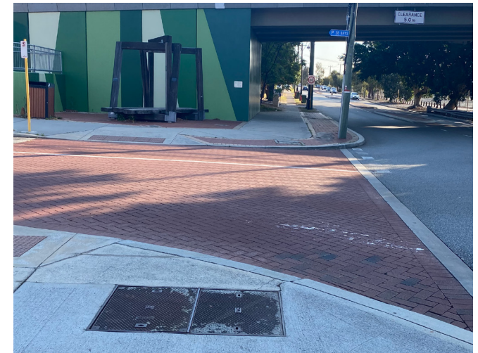
Pram ramp is slightly off the desire line, distance across is 9m
