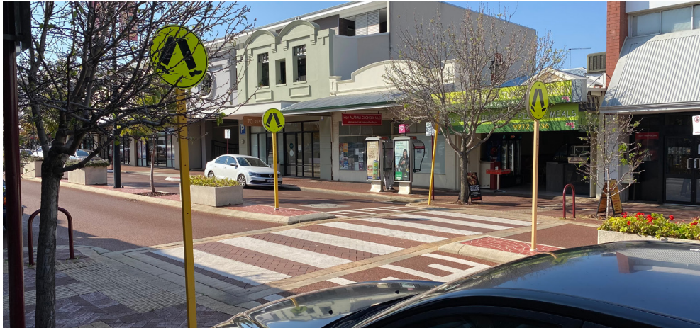
Mid-block crossing facility is step-free making it easy to cross with priority
