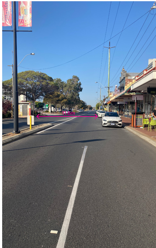
The distance between the parked car on the south and kerb-line on the north is 11.6m. There is space here for a wider footpath
