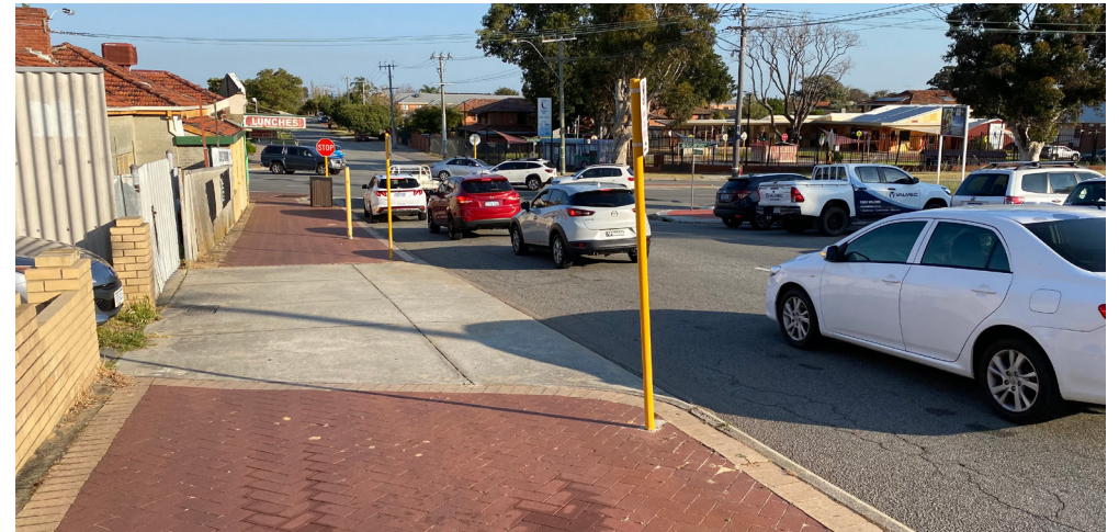
No adequate separation between traffic lane approaching Guildford Road and people walking, which creates an uncomfortable walking environment. Footpath pavement should continue over crossover.
