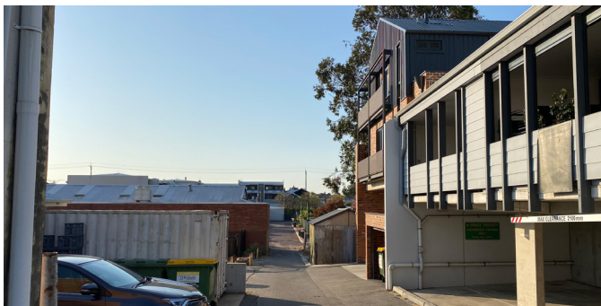
New medium-rise apartments with access to Greenslade Lane
