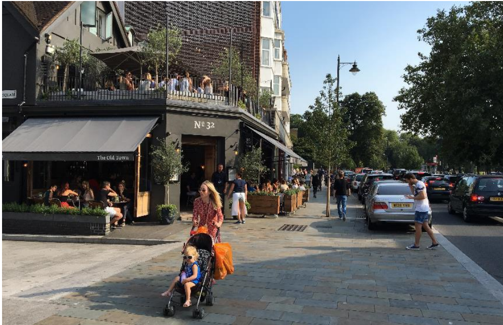
Street treatment to give people priority to cross side street entrances and maximise footpath space with inset parking bays and a level surface across footways and carriageway
