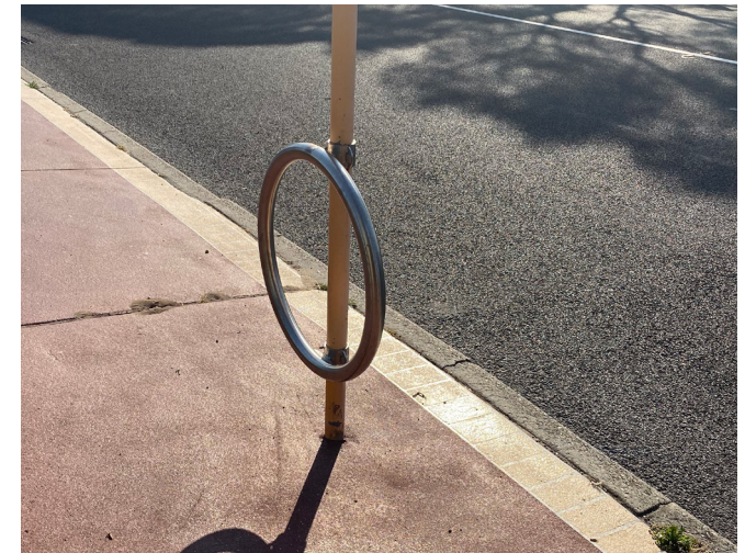
In order for bicycle parking to be accessible to all people who cycle, there must be no level differences near the parking
