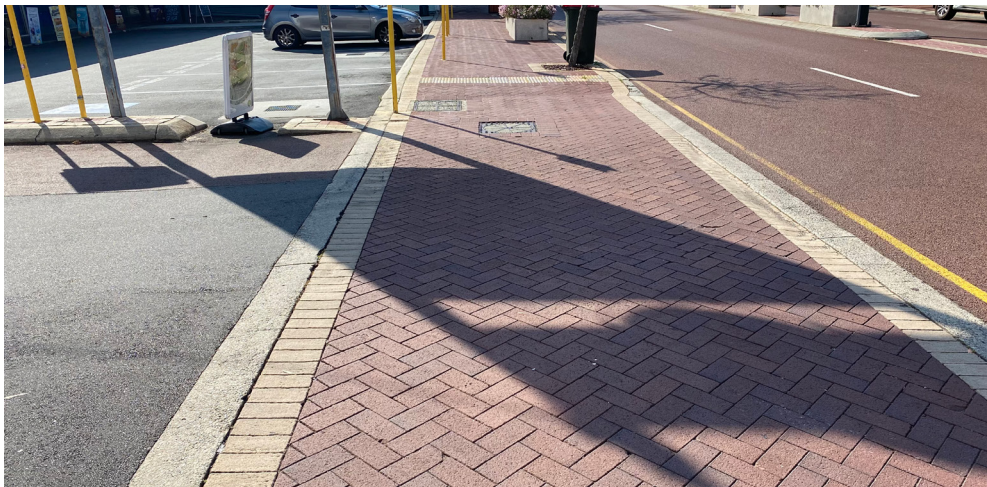
Side street entries to laneways and car parks have continuous footpath treatment reinforcing priority for people walking, but could be narrowed to make it safer
