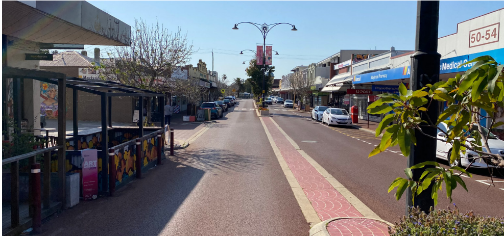
Flush median provides a form of visual narrowing of lanes that can slow vehicles
