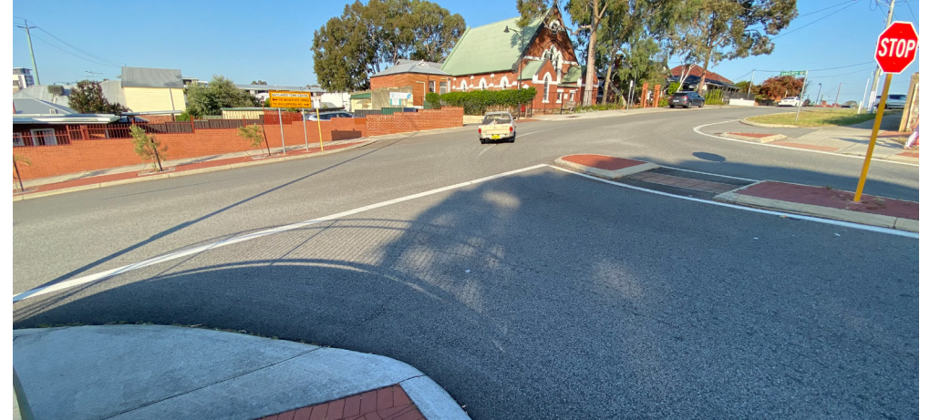
Large intersection to navigate; crossings and pram ramps to the other side of the street are non-existent, meaning fit and able cross without facilities and others travel longer down to Seventh Avenue.
