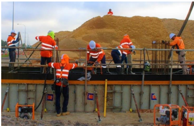
Site crew pouring the north abutment footing for the Leach Highway and Welshpool Intersection bridge
