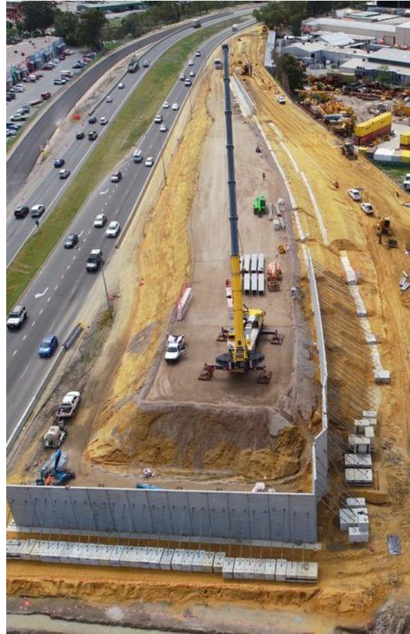
Facing north from the Leach Highway and Welshpool Road intersection, this photo shows installation of pre-cast wall panels from the crushed recycled concrete crane pad.
