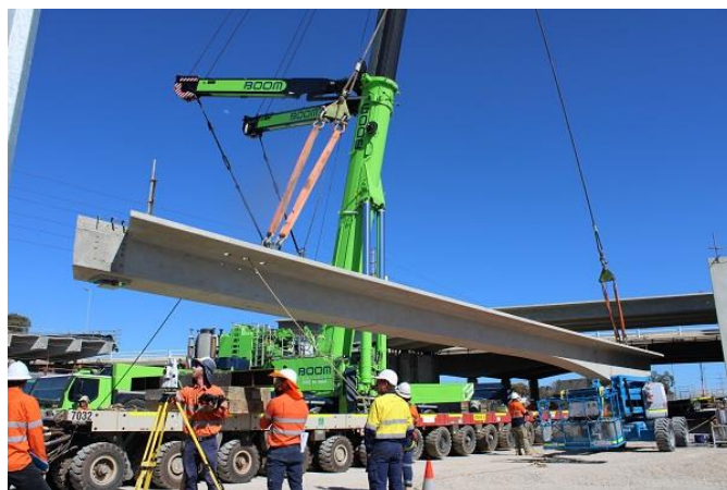
Bridge over the railway line: One of the beams being lifted for the duplicate bridge.
