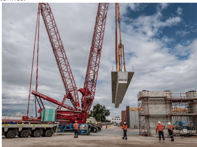
Bridge over Welshpool Road: A beam being lifted for the new Leach Highway bridge over Welshpool Road.
