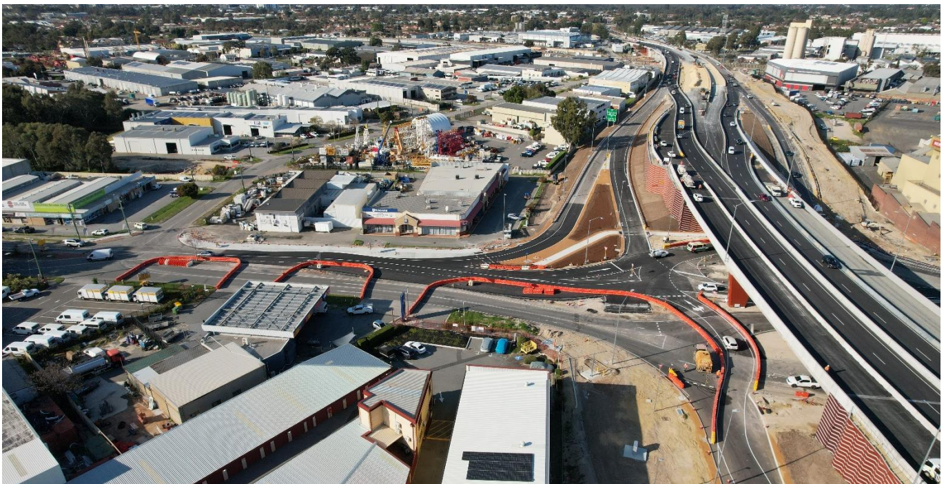
Above: Access from Welshpool Road to Leach Highway southbound open via the new ramp.
