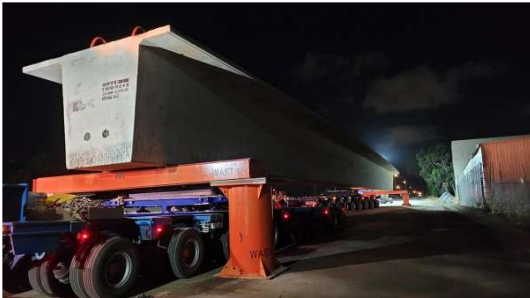
One of the beams for the Leach Highway bridge being delivered to site.
