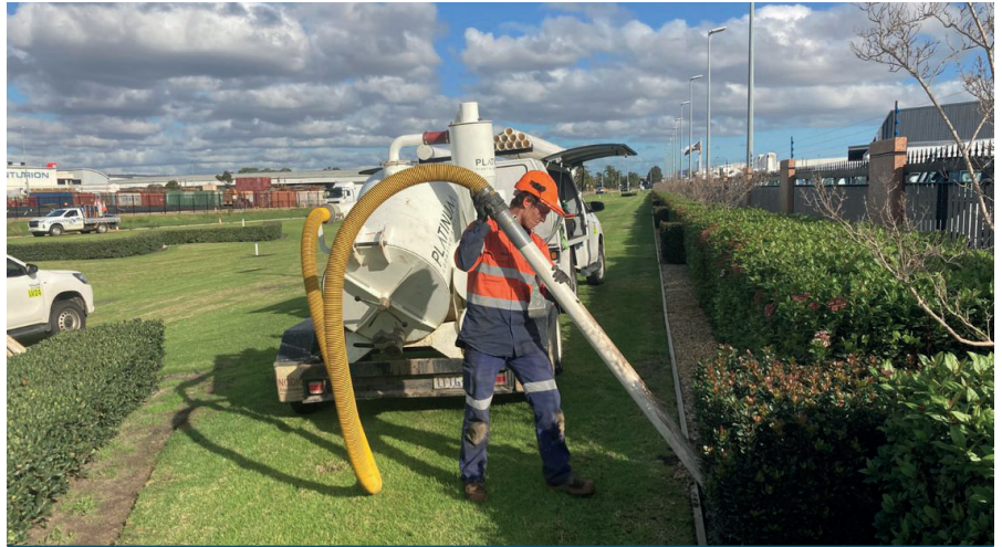
Pot-holing to identify the location of underground services.
