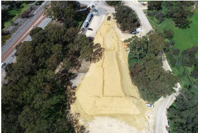
Figure 3 Drone image of work site on Heirisson Island
