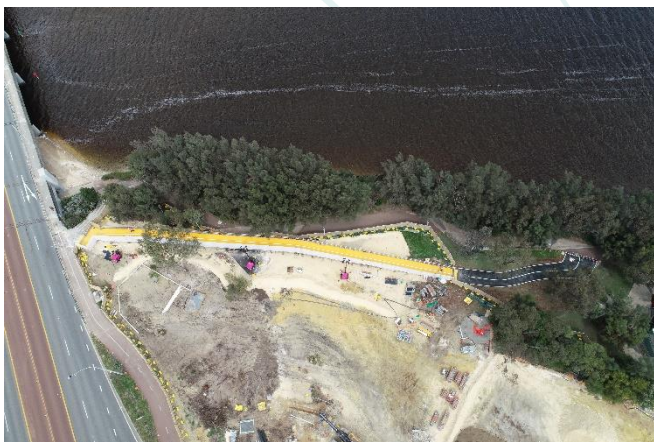
Figure 4 Drone image of work site on Point Fraser
