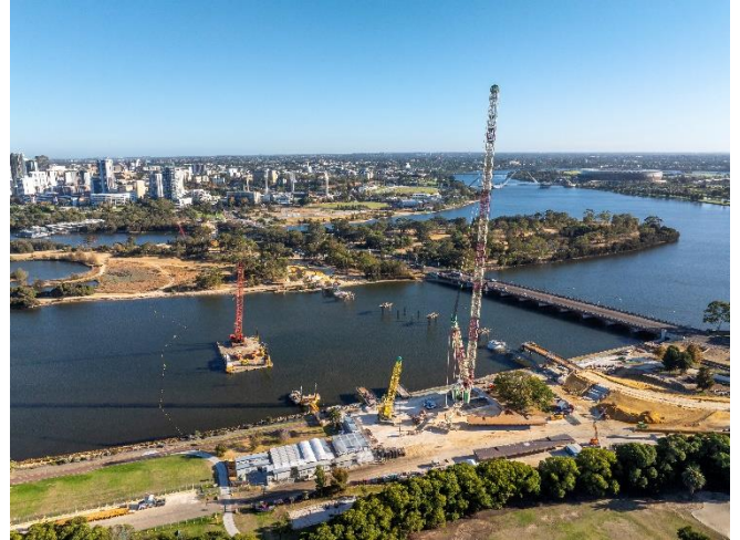
Figure 3. Large crane installed at McCallum Park site.
