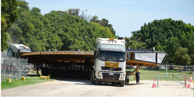
Figure 1. Bridge deck segment being delivered to site.
