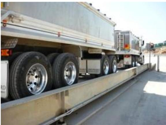
Some weighbridges have multiple decks allowing the vehicle's axle groups to be weighed simultaneously and software systems that provide the driver with printed dockets showing these weights.
