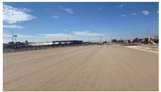
Figure 4 Trimmed and compacted CRC on the Armadale Road North Lake Road Bridge Project
