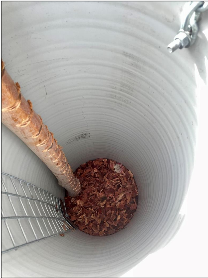
Wood Chips, ladder and Sacrificial post.
