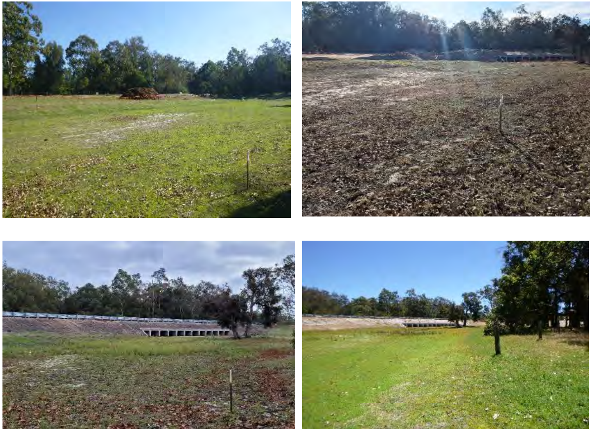
Plate 4. Ongoing construction works at BSM-S-PI-2 from photopoint monitoring locations. Top left: Q2 monitoring 2023, top right: Q2 2024, bottom left: Q2 2025, bottom right: Q4 2025.
