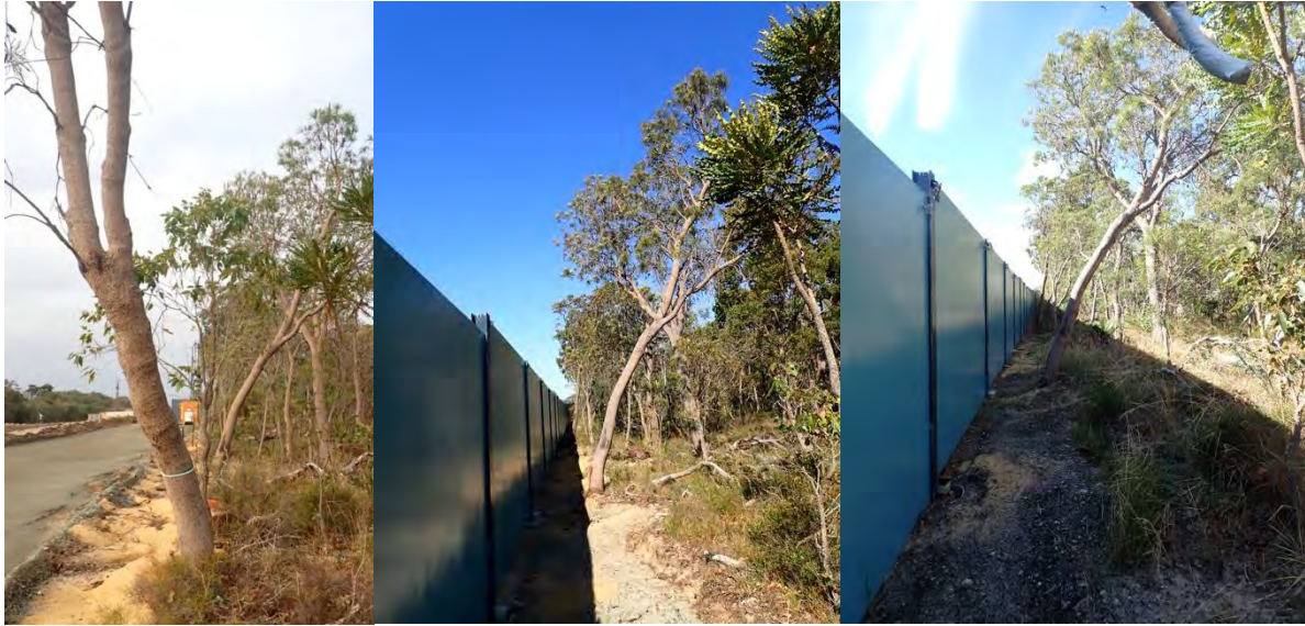
Plate 16. BW-S-PI-8_P01 autumn 24 and spring 24. Note that the Banksia in the foreground had to be removed for the installation of the sound wall.
