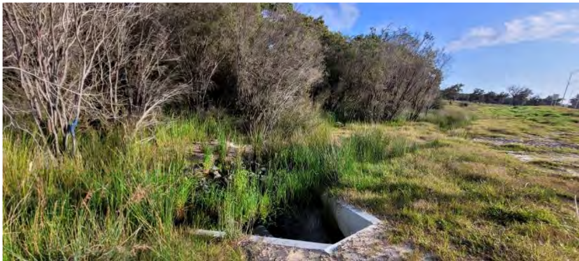
Plate 5. Infrastructure (culvert / run-off drain) into receiving wetland UFI-1117
