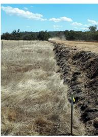
Photograph 4: Pegging of clearing line to demarcate disturbance boundary
