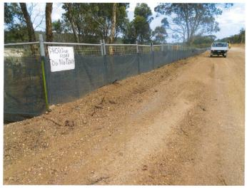
Photograph 1: Fencing to demarcate and protect TEC during construction
