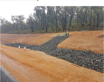
Photograph 5: Gross pollutant trap, incorporating rock protection, at the inflow point to the culvert that drains into the TEC
