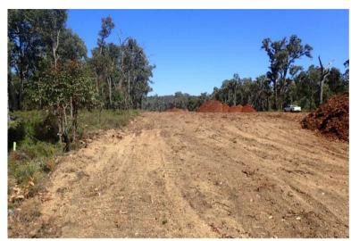
Photograph 3: Pegging of clearing line (on left of photo) to demarcate disturbance boundary
