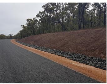
Photograph 6: Longitudinal drain scour protection
