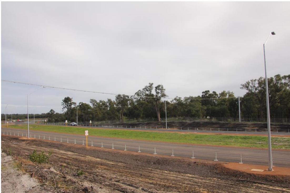
Plate 1 Rope bridge layout and components
