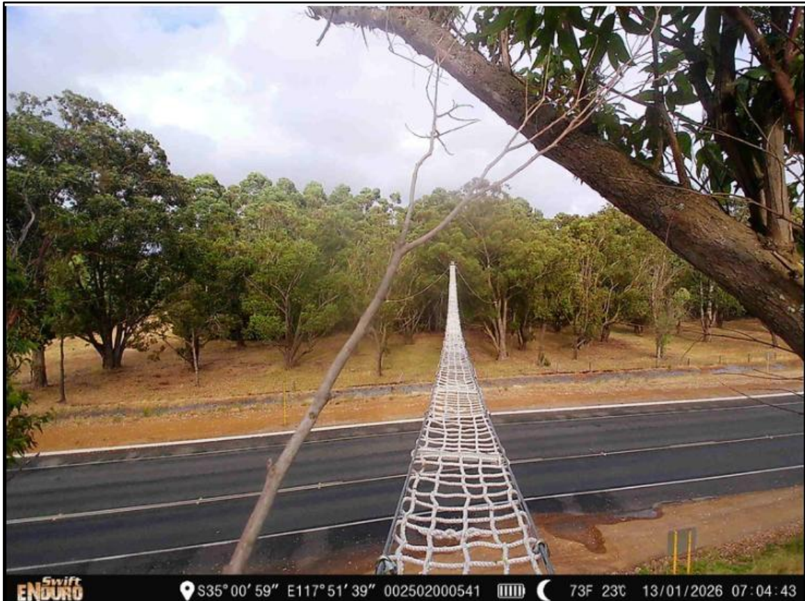
Photo 2b. Fauna rope bridge across Hanrahan Road (looking west across from bridge, camera 2).
