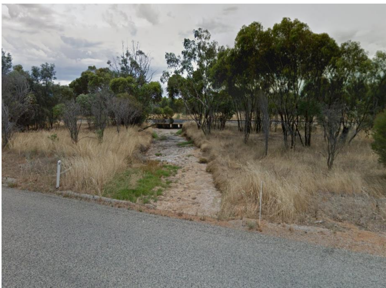
Plate 2: Looking downstream, LHS Bindoon Moora Road
