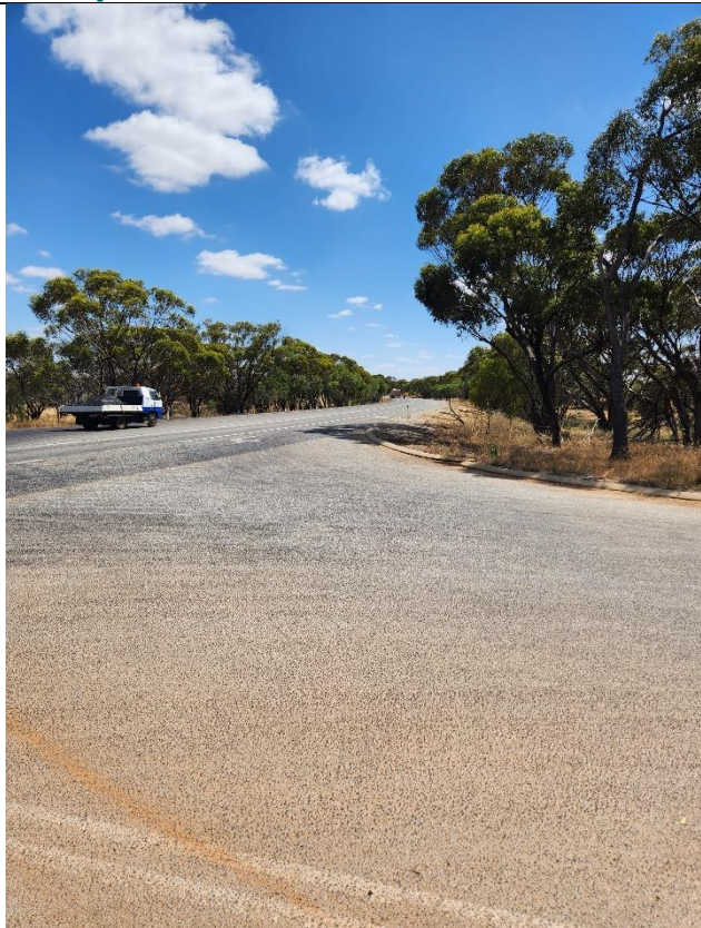
Photo 1: Quellington Road and GEH intersection looking West
