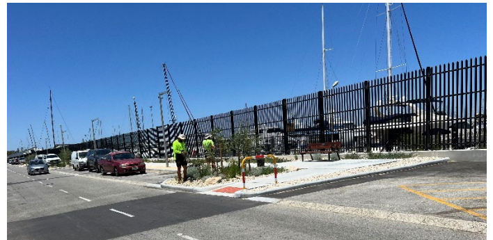
Bithuwanda Fenceworks installation under way
