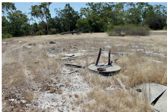
IMG_0142 .....400398 mE 6484323 mN Concrete floor 8 m x 3m . Asbestos sheets and two septic tanks.
