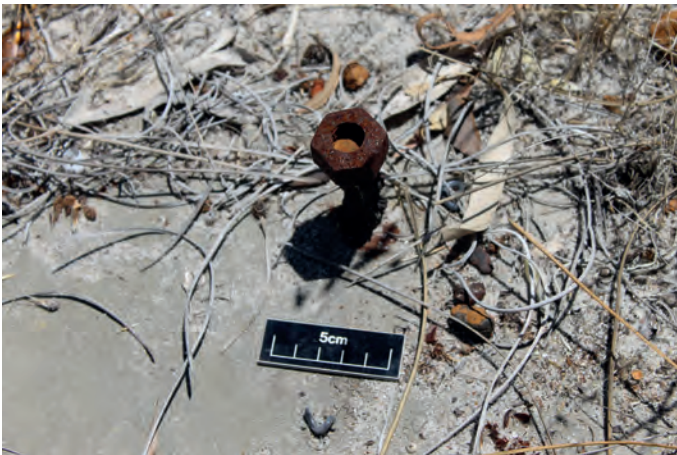
IMG_0109 .....400387 mE 6484197 mN Steel bolt/stud for fixing wooden wall bearers.
