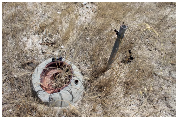
IMG_0144 .....400393 mE 6484356 mN House water drain (terracotta) with galvanised steel pipe.
