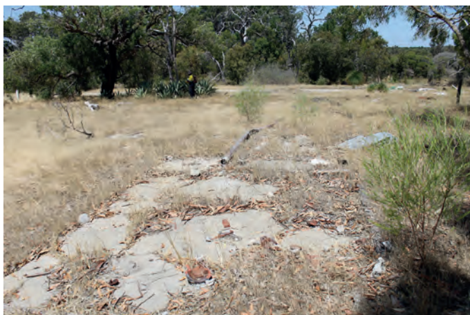
IMG_0116 .....400399 mE 6484253 mN Concrete floor/toilet slab. Wooden floor joists bolted to floor. Note terracotta pipe.
