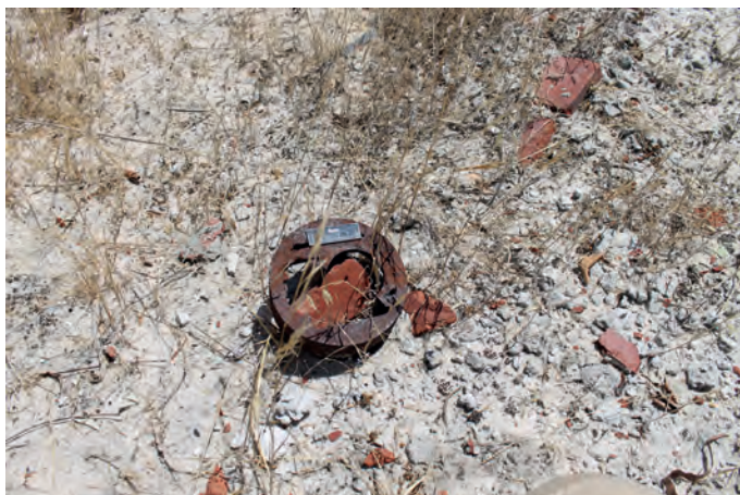
IMG_0143 .....400393 mE 6484356 mN House water drain (terracotta) and cast iron drain cover
