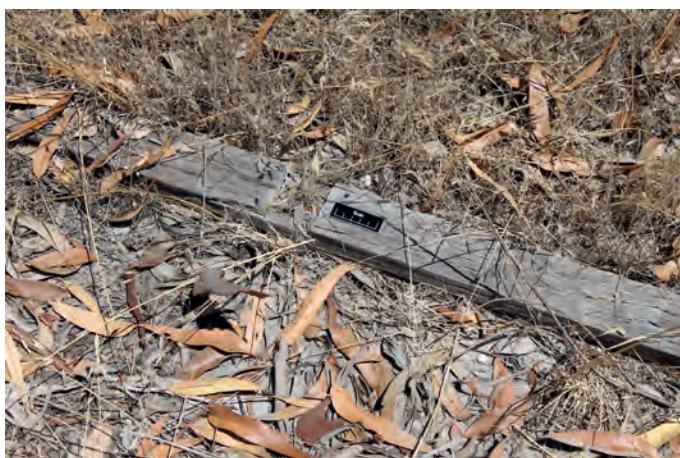
IMG_0118 .....400399 mE 6484253 mN Close view of wooden joist with trenching for wooden verti- cal studs.
