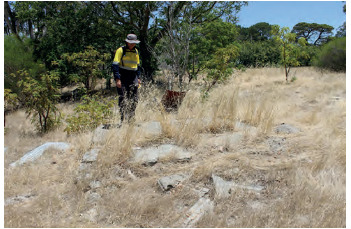
IMG_0099 .....400377 mE 6484137 mN Concrete foundation measuring 3 m x 4 m with Darren Cooper. Note asbestos sheeting.
