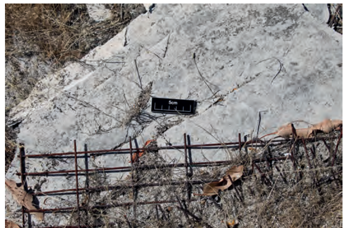
IMG_0163 .....400148 mE 6484487 mN Concrete floor with steel mesh
