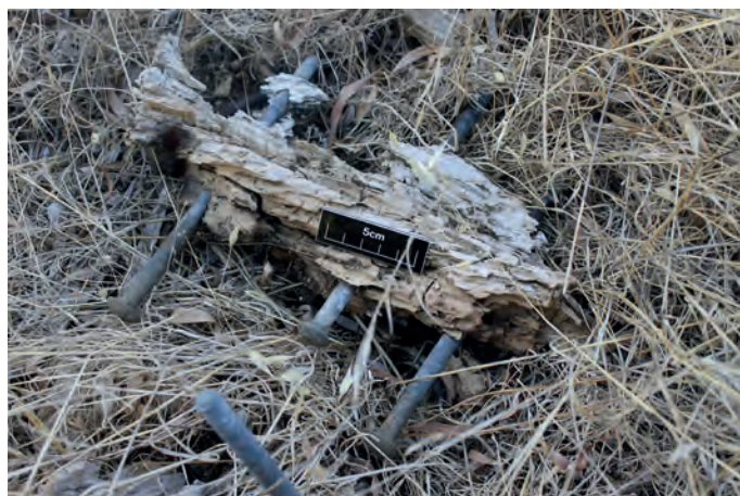
IMG_0174 .....400333 mE 6484038 mN View of large galvanised bullet head bolts.
