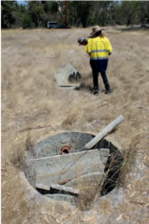
IMG_0085 .....400304 mE 6484189 mN Septic tank and leach drain with S. Kendall and D. Cooper.
