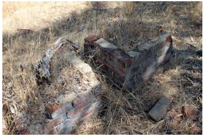
IMG_0041 .....400156 mE 6483968 mN 2 red brick features - 65 cm x 70 cm x 45 cm. Five courses of bricks high, set on concrete blocks, rendered
