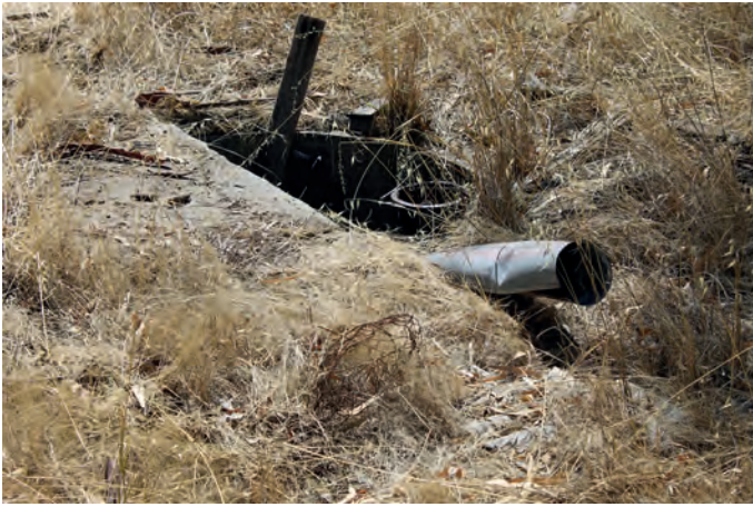
IMG_0038 .....400167 mE 6483958 mN Open septic tank with down pipe inserted
