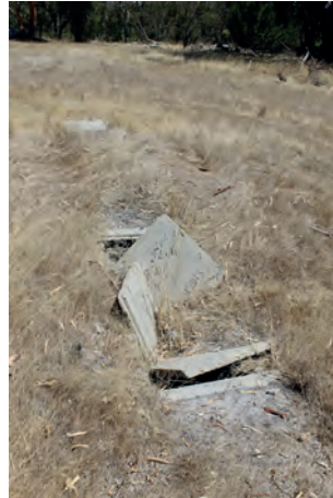
IMG_0086 .....400304 mE 6484189 mN Close view of leach drain.
