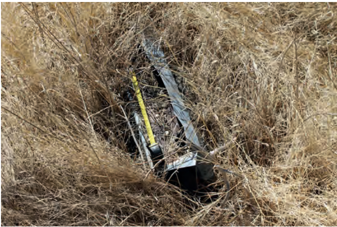
IMG_0028 .....400148 mE 6483882 mN Tin gutter end with downpipe
