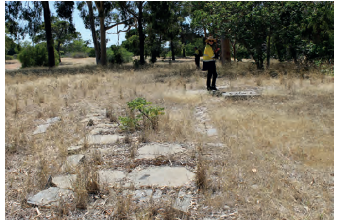
IMG_0070 .....400175 mE 6484040 mN Concrete Path leading to three heavy duty foundations. With S. Kendall and D. Cooper. Looking east.
