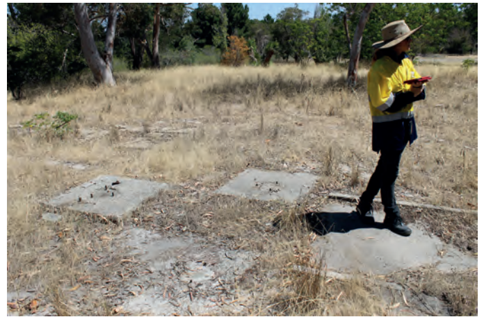
IMG_0072 .....400175 mE 6484040 mN S. Kendall standing on well-formed concrete 'slipway'. Note heavy-duty foundations in foreground.
