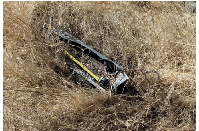
IMG_0029 .....400148 mE 6483882 mN Tin gutter end with downpipe
