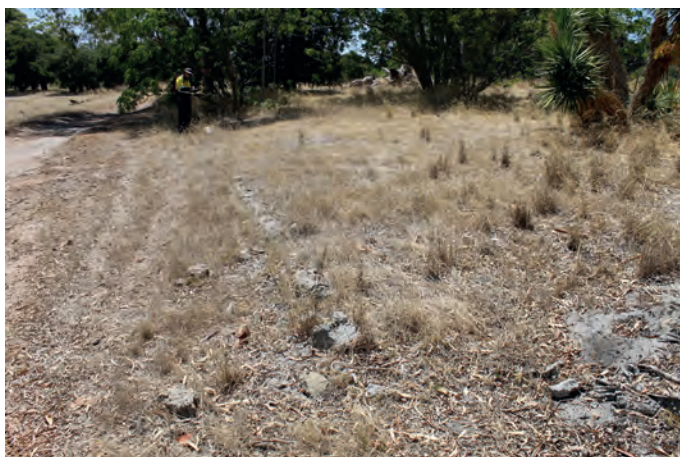
IMG_0077 ..... mE mN Concrete retaining wall.
