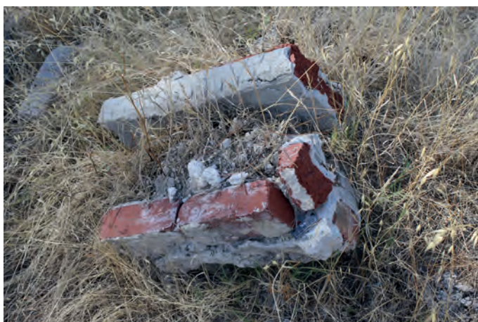
IMG_0018 .....400143 mE 6483918 mN Brick Foundation - close view
