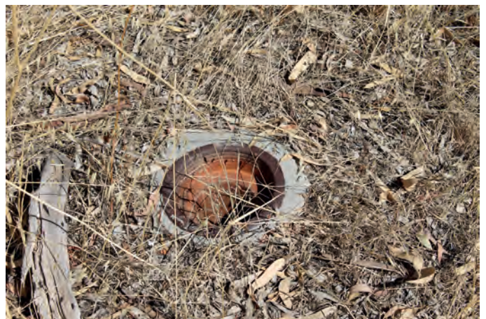
IMG_0037 .....400167 mE 6483958 mN Terracotta house floor drain
