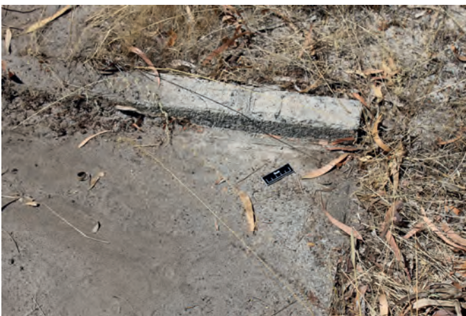
IMG_0073 .....400175 mE 6484040 mN Close view of well-formed concrete 'slipway'. Note joins.
