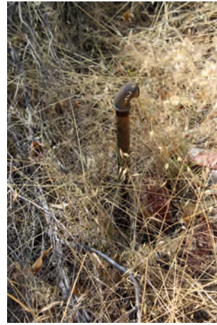
IMG_0058 .....400192 mE 6483995 mN Galvanised Steel Water Pipe
