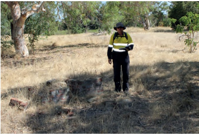
IMG_0040 .....400156 mE 6483968 mN 2 red brick features - 65 cm x 70 cm x 45 cm. Five courses of bricks high, set on concrete blocks, rendered
