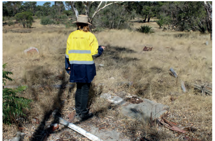
IMG_0035 .....400167 mE 6483958 mN Concrete pad - Toilet block, 2 septic tanks (both with bees), drain pipe; timber footing, 5 m x 6 m
