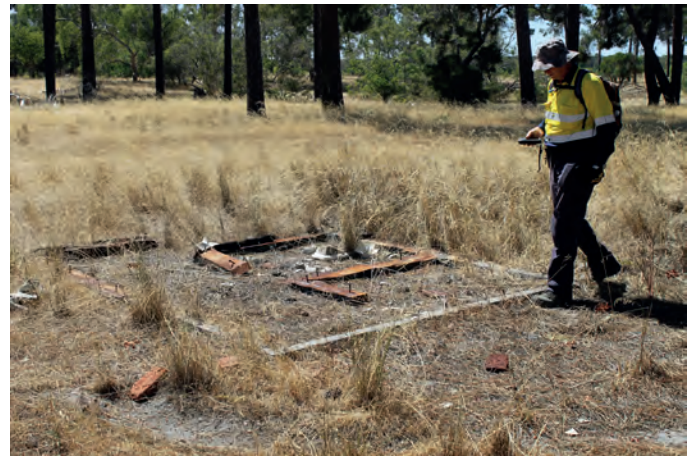
IMG_0060 .....400027 mE 6484022 mN Concrete toilet block. Note the used of studs for wood/ asbestos sheet walls and tin termite barriers. With Darren Cooper.
