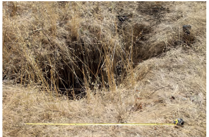
IMG_0011 .....400143 mE 6483918 mN Hidden open septic tank. Note grass coverage.
