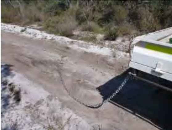
Plate 1 Heavy chain rig designed to clear track
