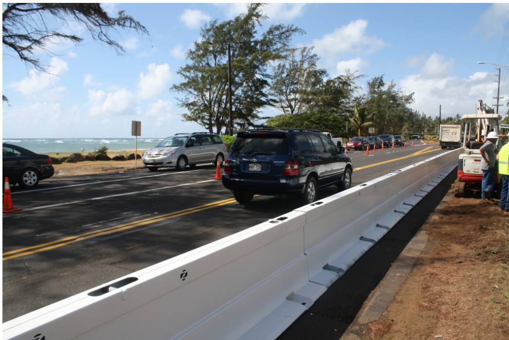
Photograph of ZoneGuard installation
