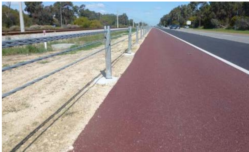
Photograph of Sentryline II wire rope safety barrier installation.
