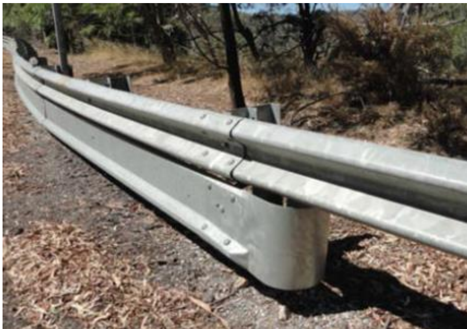
Photograph of the Rolled End Section of the HIASA Rail
