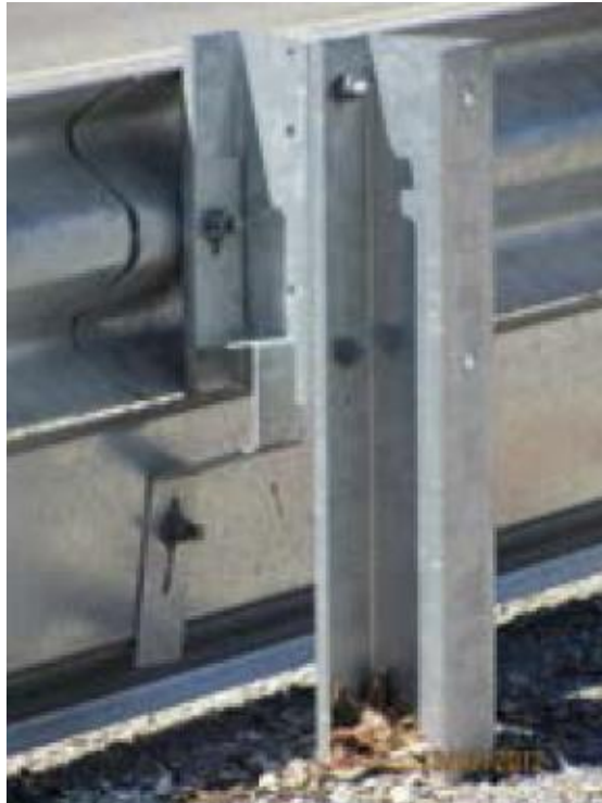
Photograph of the HIASA Rail connection to W-Beam
