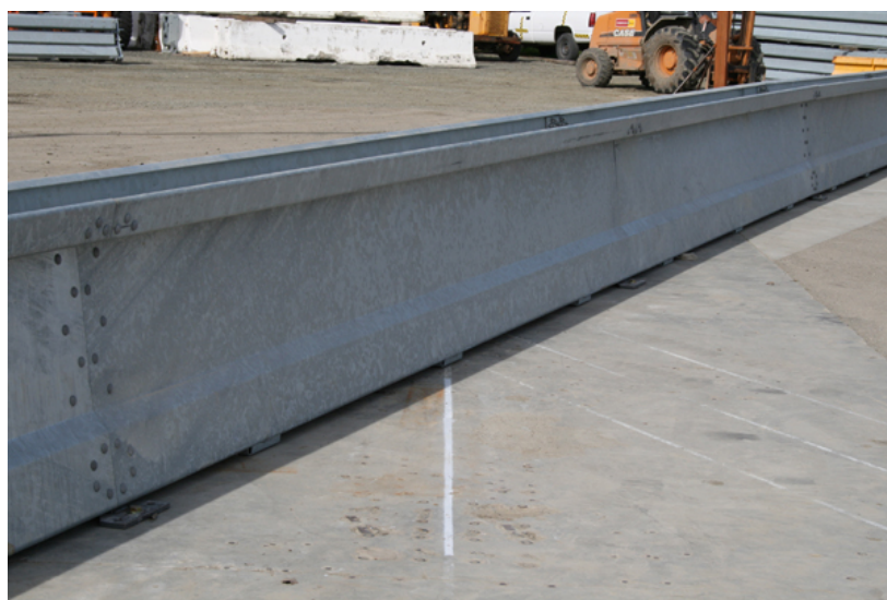
Photograph from BarrierGuard MDS installed (showing T-Top section)
