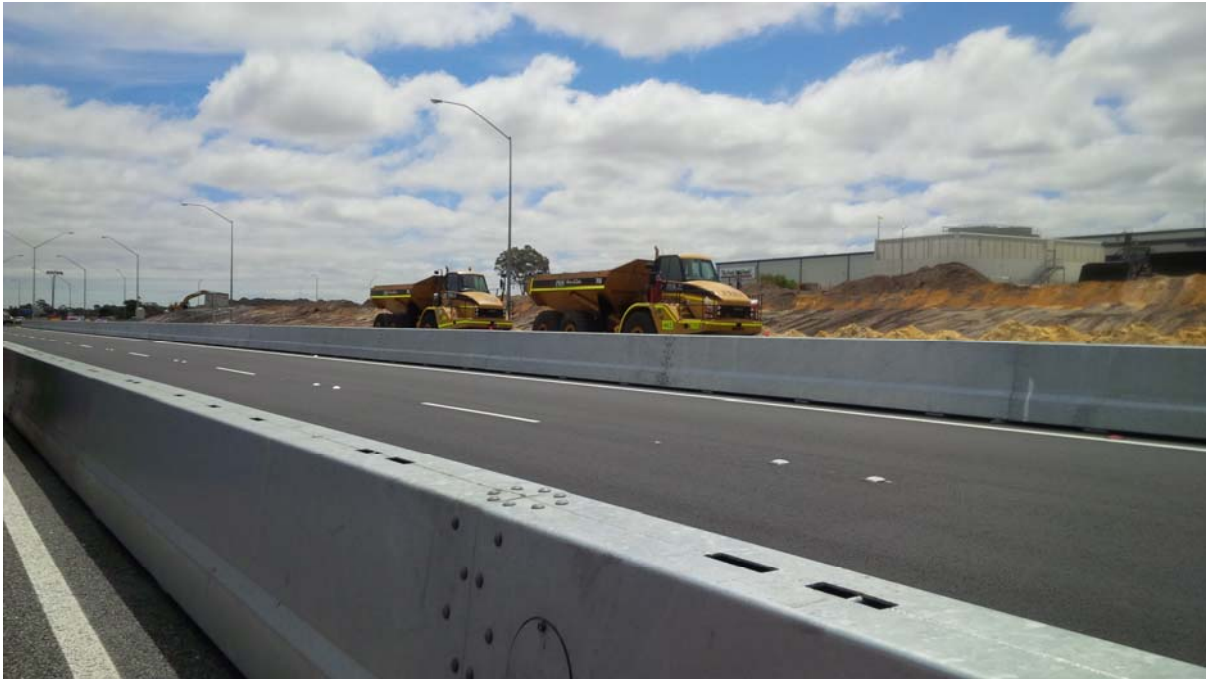
Photograph from BarrierGuard 800 installation
