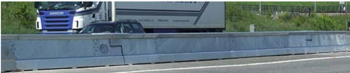
Photograph of BarrierGuard 800 Gate installation
