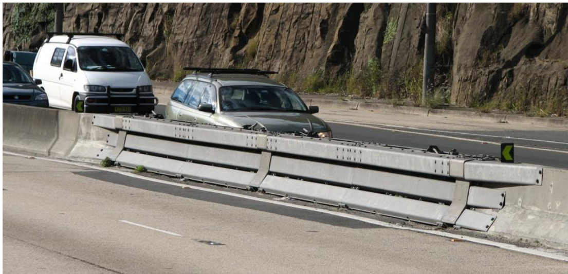
Photograph of ArmorGuard Gate installation
