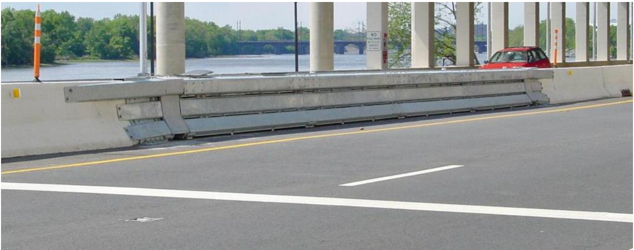
Photograph of ArmorGuard Gate installation
