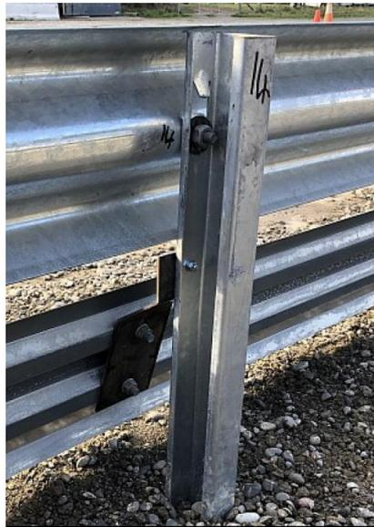
Rear view of RiderPro connected to Sentry W-Beam
