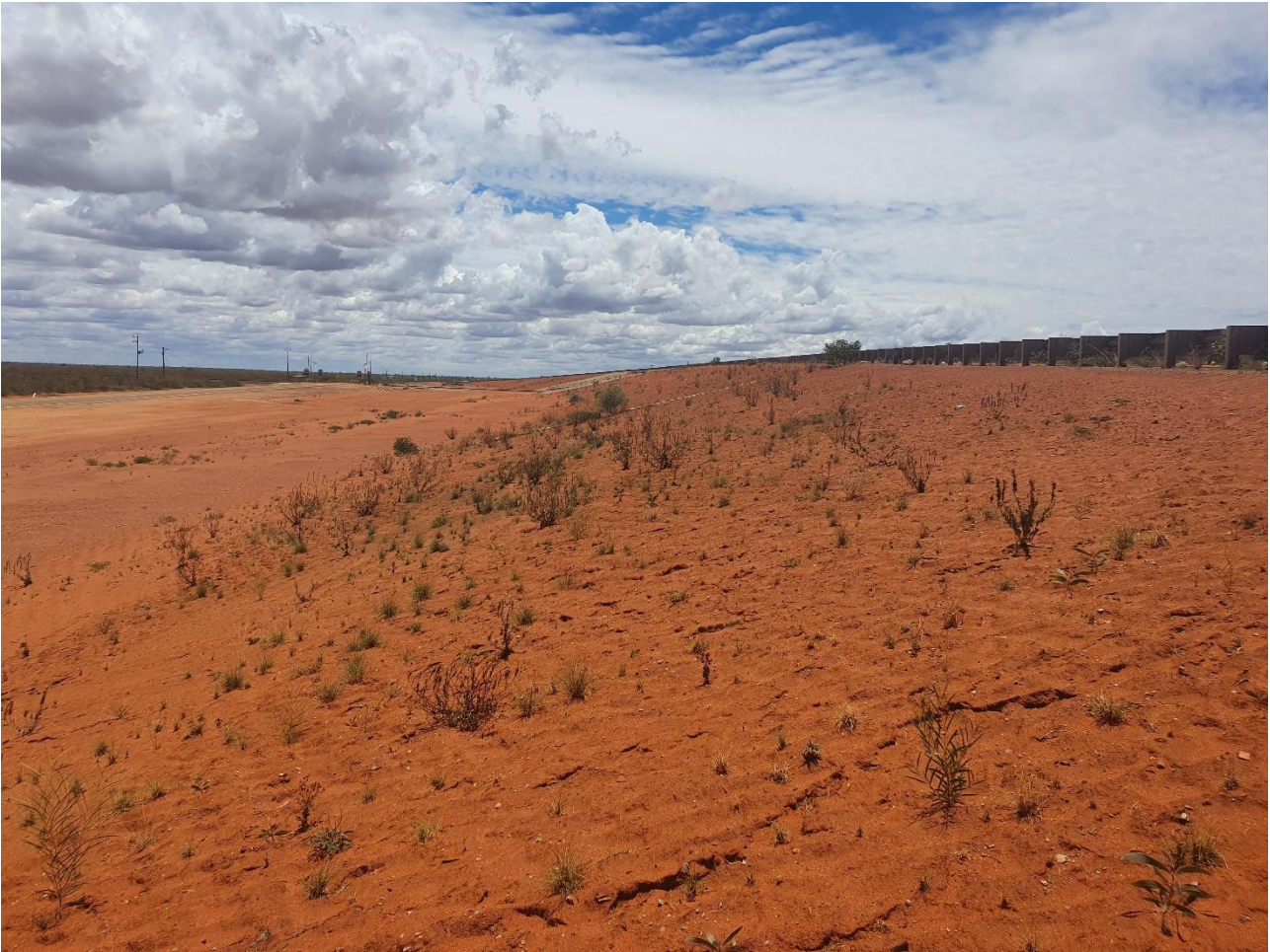
Figure 3: Post Rip and Respread of Great Northern Highway
