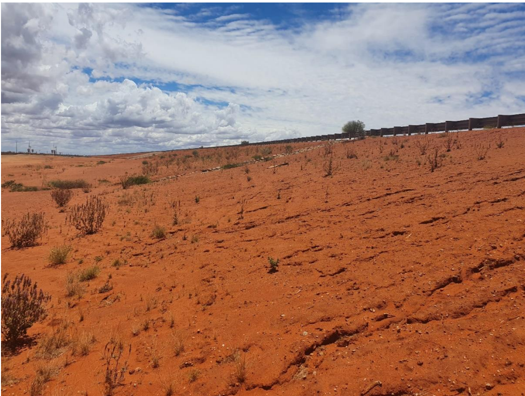
Figure 2: Post Rip and Respread of Great Northern Highway
