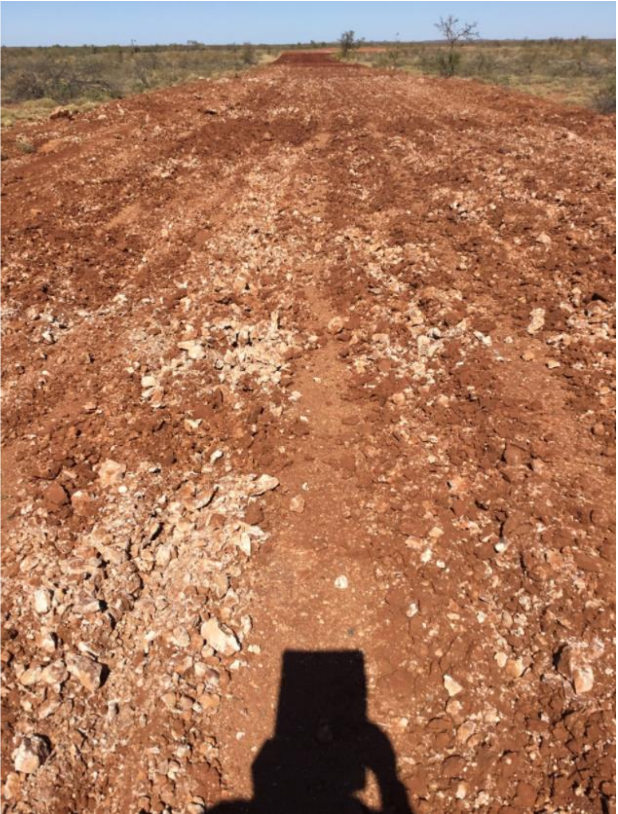
Figure 1: Rip and Respread at NWCH pit
