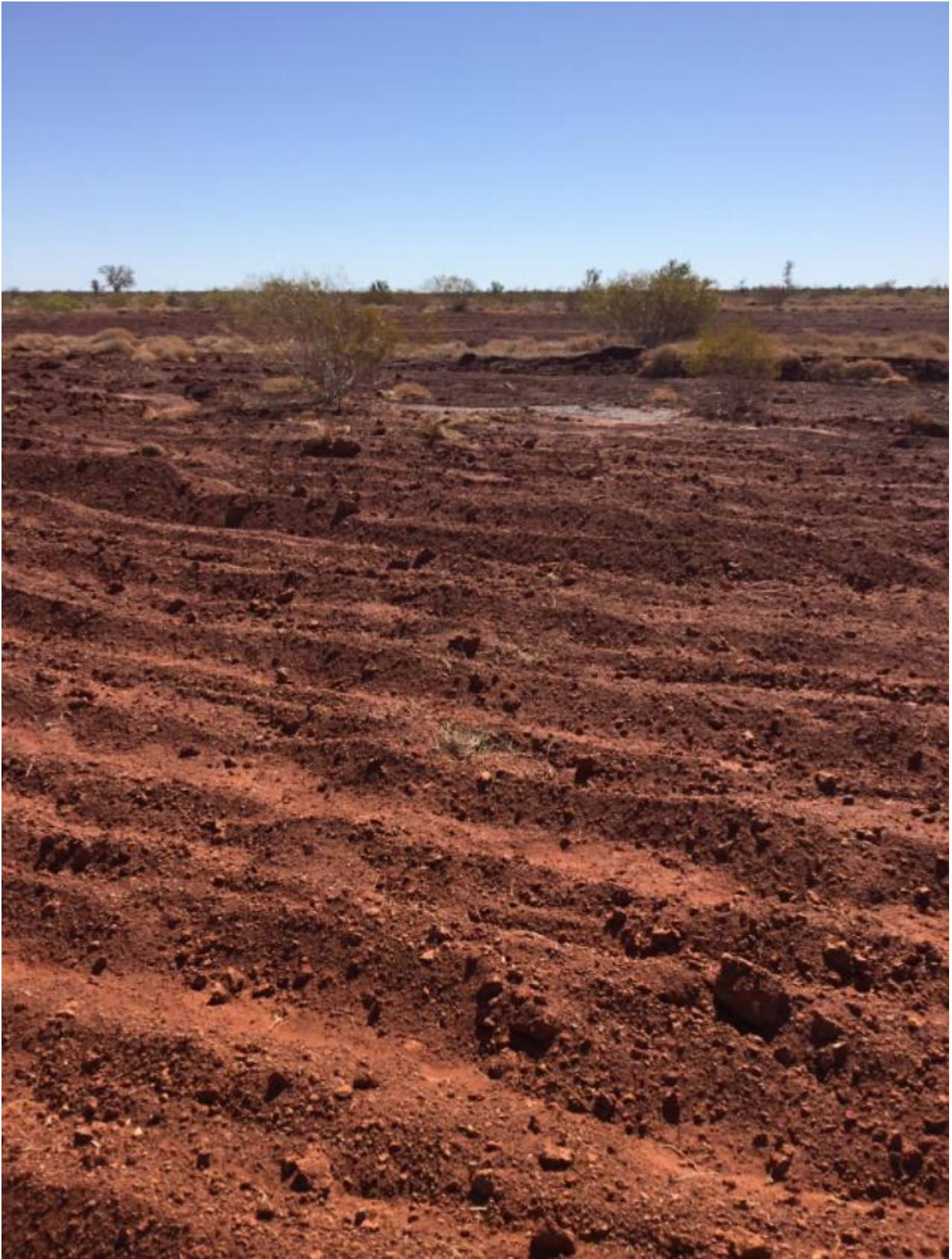
Figure 2: Rip and Respread at Onslow Road legacy pits
