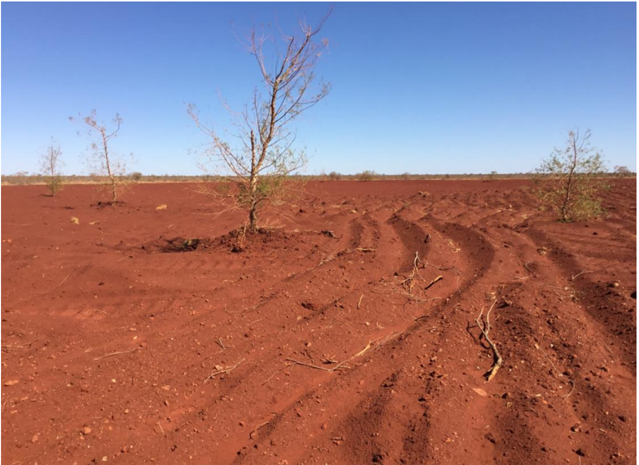
Figure 1: Rip and Respread at Onslow Road Legacy pits
