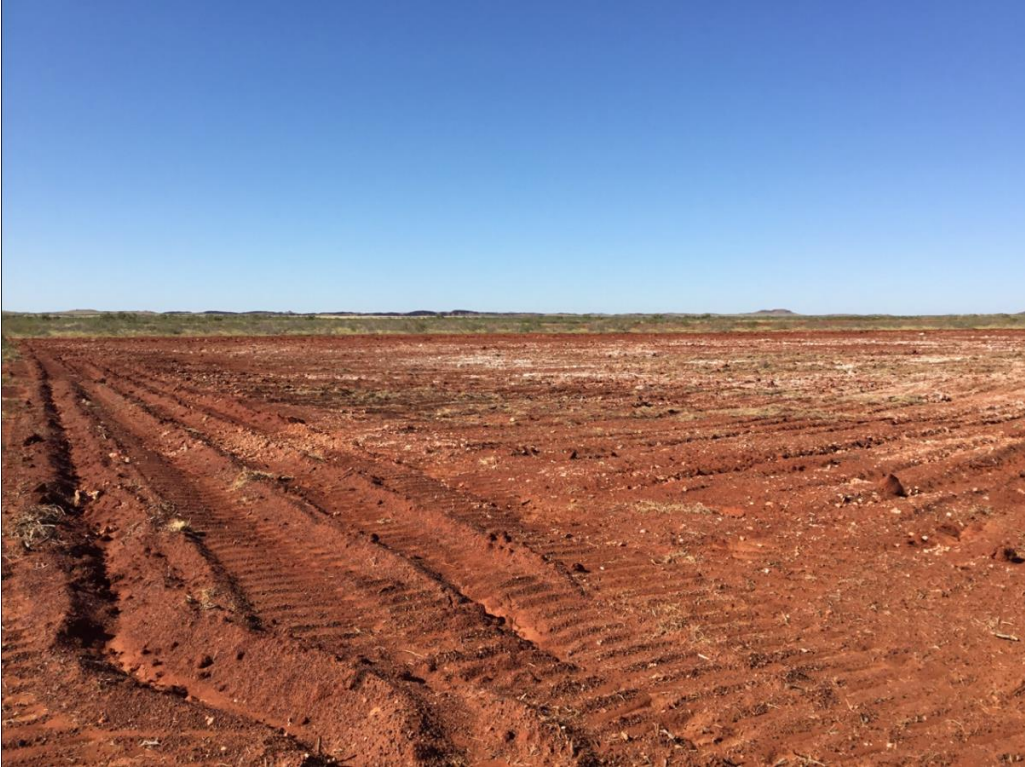
Figure 1: Ripping and Respread at Madigan Rd
