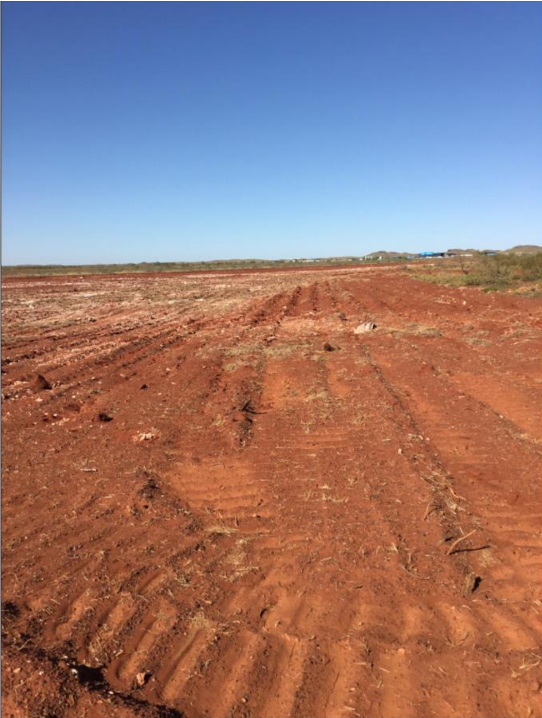
Figure 2: Ripping and Respread at Madigan Rd
