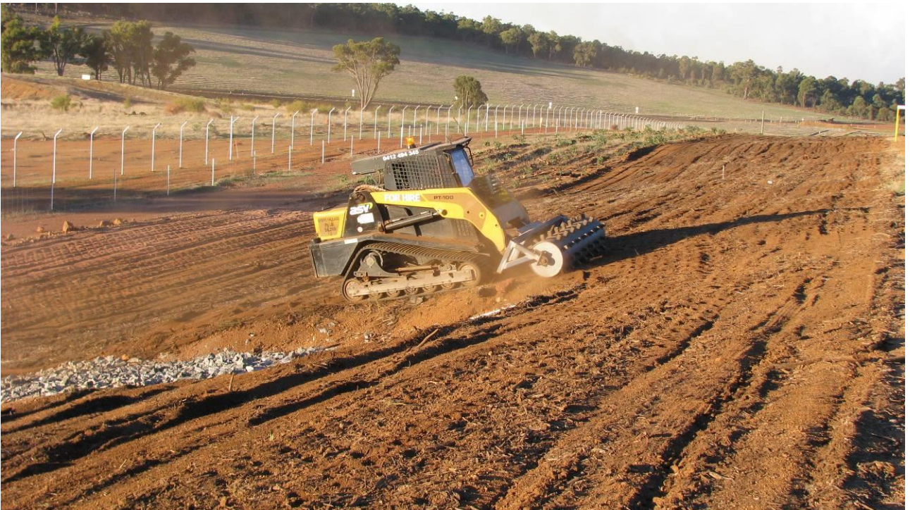
Figure 2. Batters prepared prior to direct seeding/planting in July 2012.
